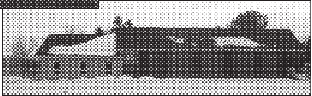
Present building showing the addition to the front.
