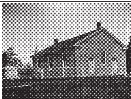
Original building at Jordan, Ontario
