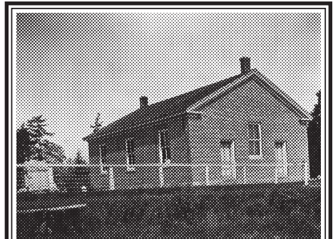
Original building at Jordan, Ontario
