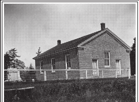
Original building at Jordan, Ontario
