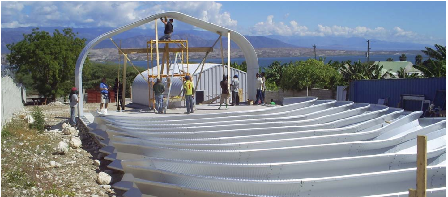
Orphanage building assembly begins
