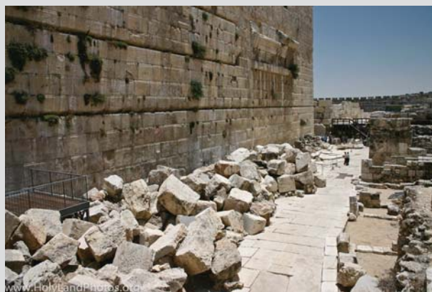
First Century shops and street below Robinson's Arch at the Jerusalem Temple Western Wall in fulfillment of Jesus' words: "Do you see these stones? Not one stone will be left upon another which will not be torn down" Mark 13:2 "I tell you, if these become silent the stones will cry out!" Luke 19:40 Photo: http://holylandphotos.org/
